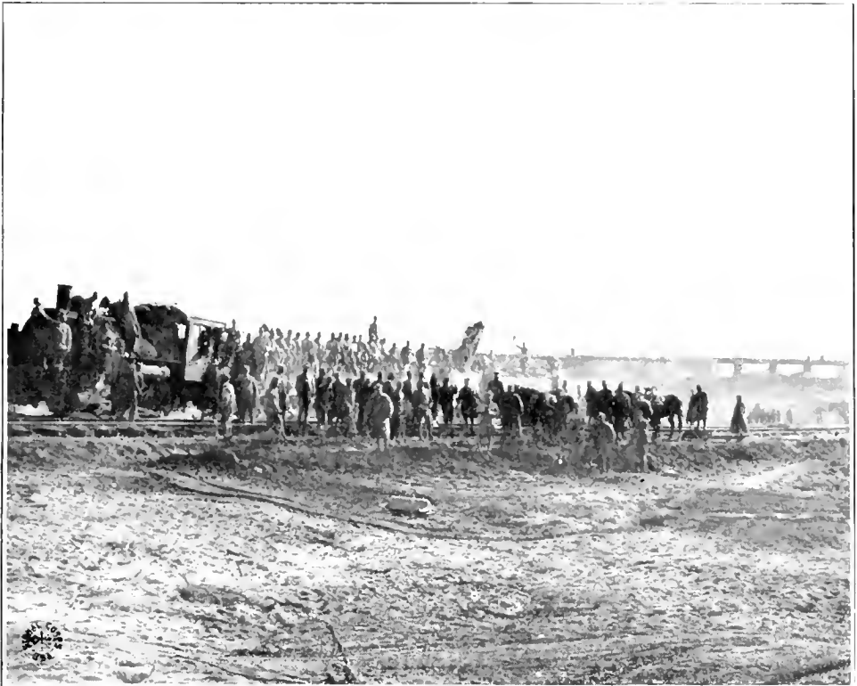
ITALIAN TROOPS AT WORK ON THE SERMOISE END OF THE NEVERS RAILROAD CUT-OFF, NOVEMBER 20, 1918
